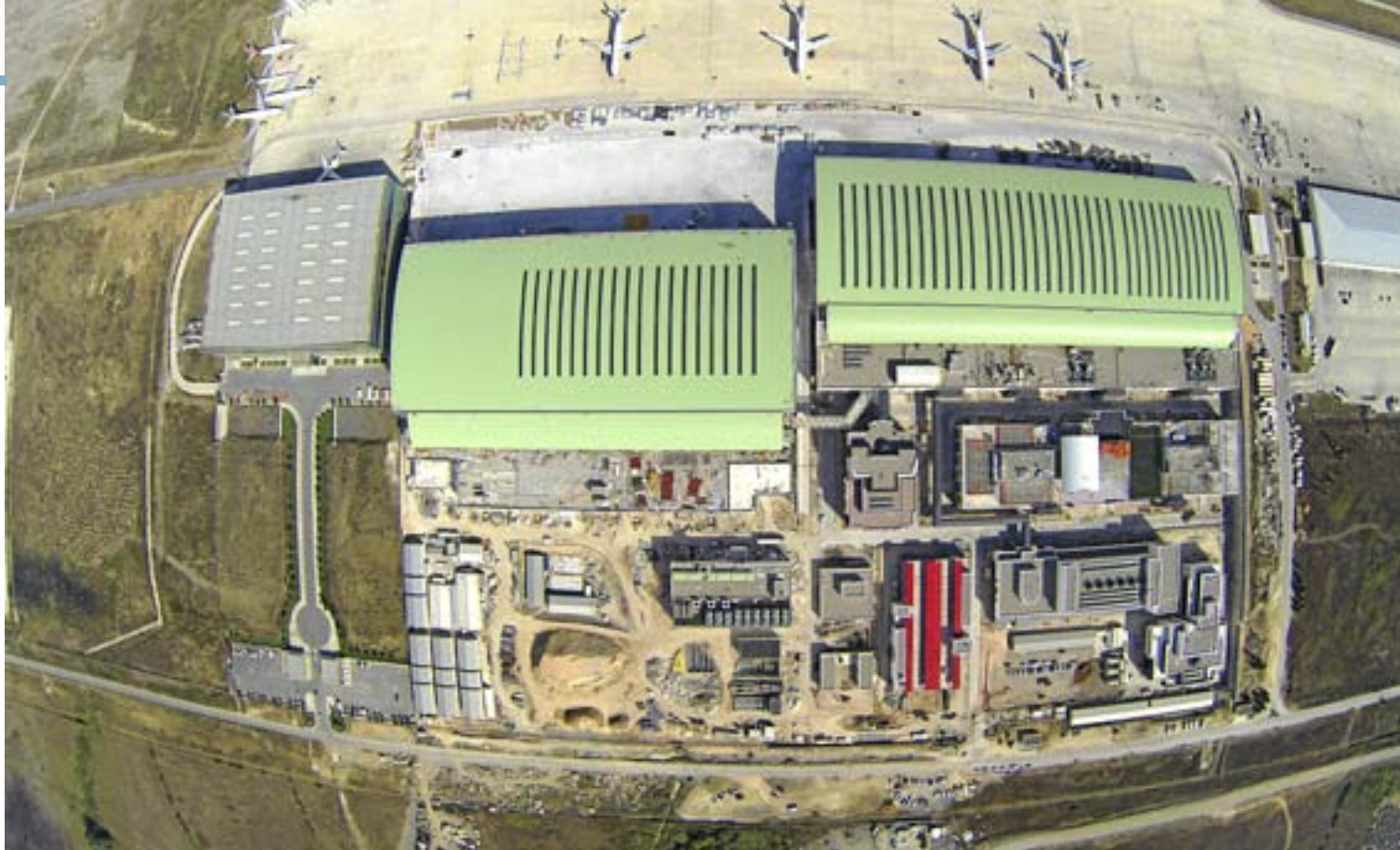
▲ A new facility is under construction at Habom.
